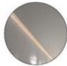
Open Ceiling Painted Light Blue
